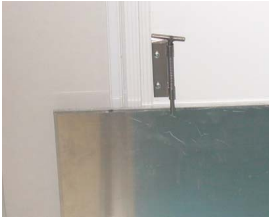
Figure 44: Patient Door Inner and Outer Floor Transition Plates Up and Locked
