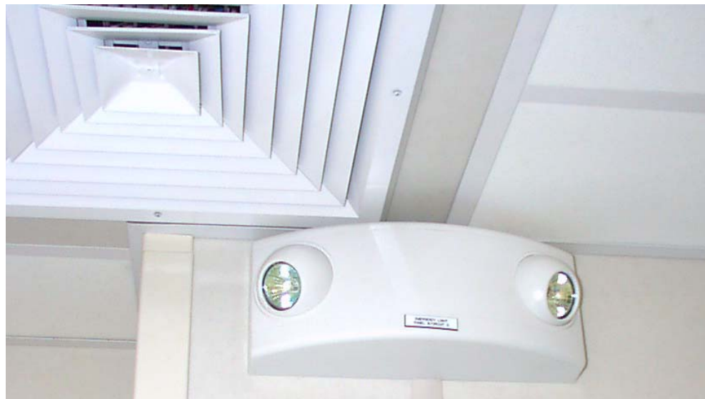
Figure 59: Emergency Dual Beam Lighting (Typical)
