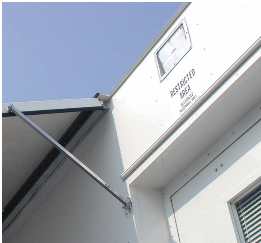
Figure 62: Staff Door Lighting
