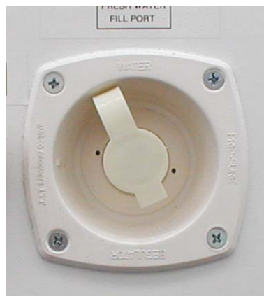
Figure 51: Humidifier External Water Connection
