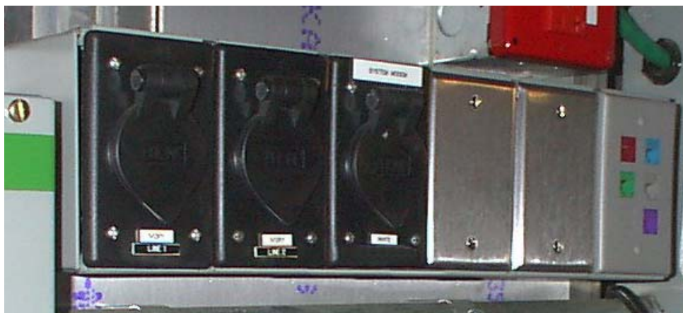
Figure 25: Phone and Data Line Connections (Typical)
