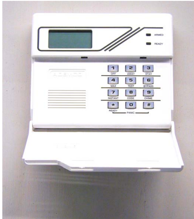
Figure 56: Intrusion Alarm Keypad
