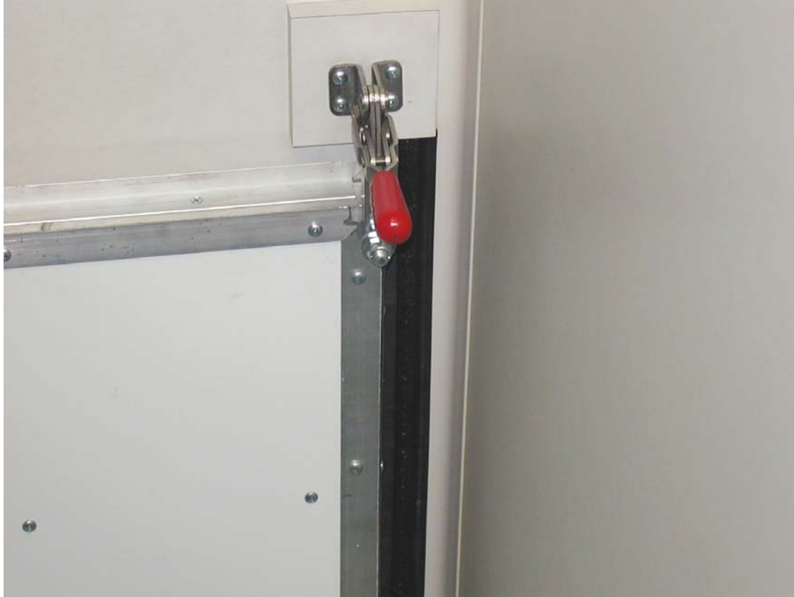
Figure 21: Slide-out Floor and Transport Latch (Transport Mode)
