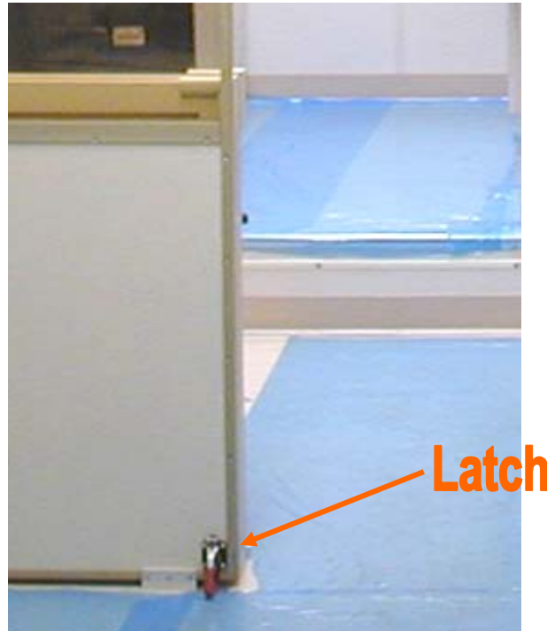
Figure 41: Procedure Room Sliding Door Latch
