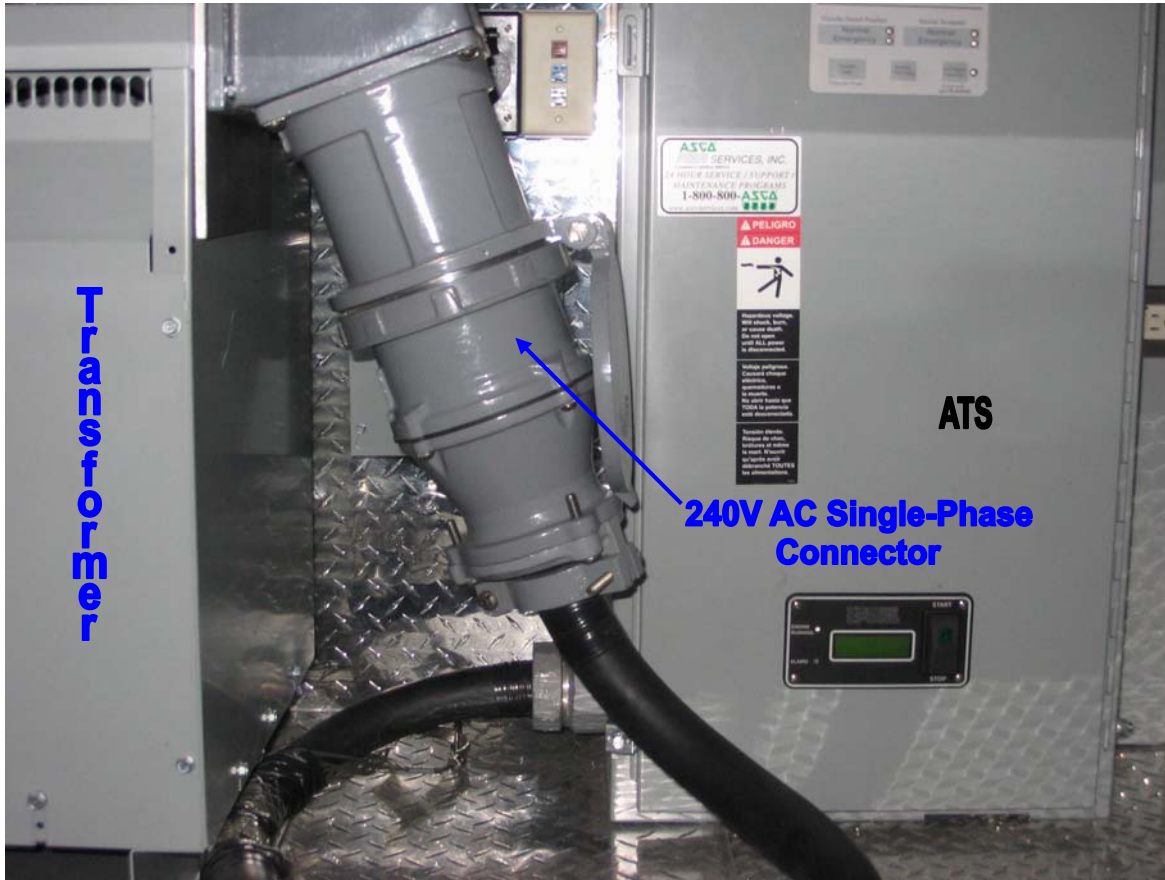
Figure 14: Automatic Transfer Switch (ATS)
