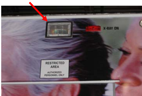
Staff Door Entry Light & X-ray on Light
