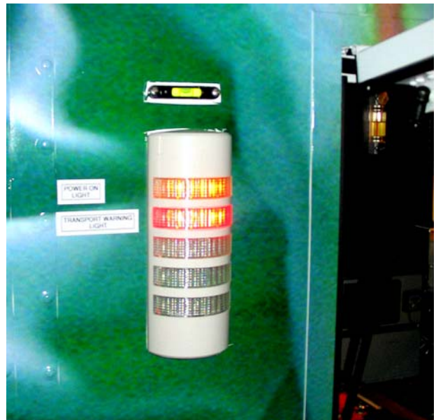
Figure 37: Power Indicator Light
