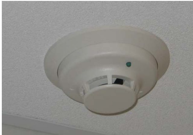
Figure 17: Smoke Detector
