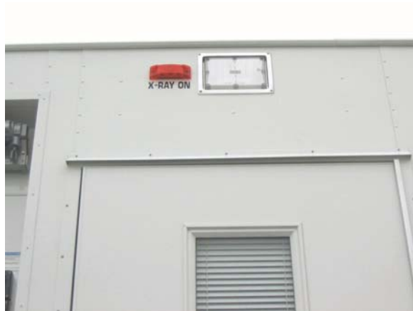
Figure 45: Staff Door Lighting
